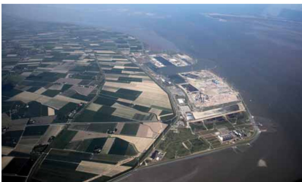
Aerial view of Eemshaven
